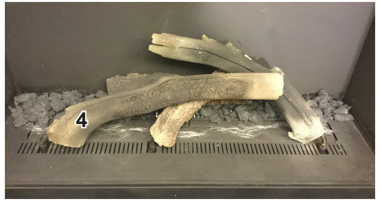
Slide block 4 (with holes) on the flexible burners
